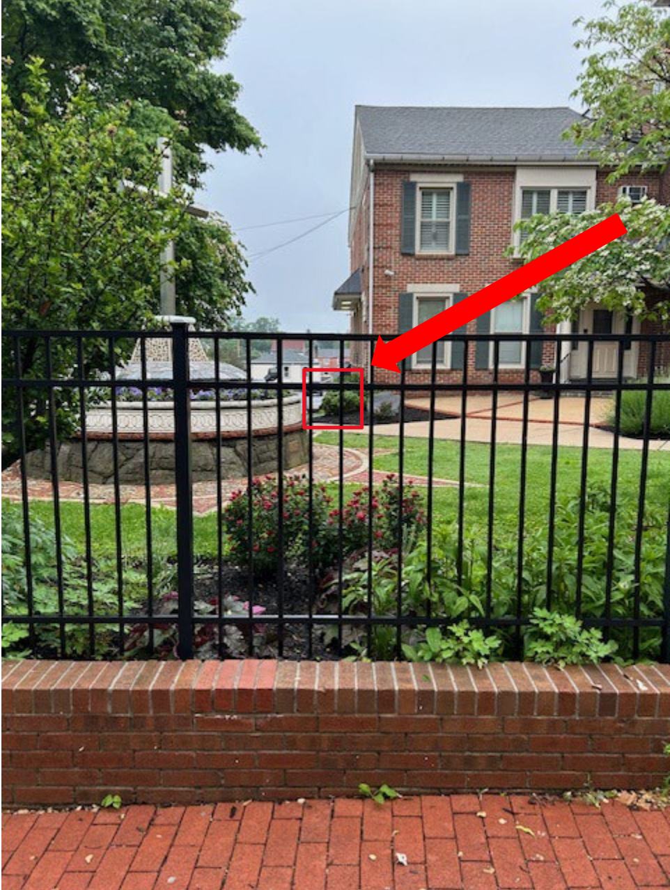
View of AC unit location from Gay Street
