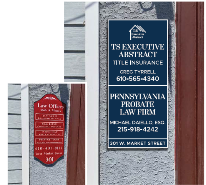
The existing building sign will be removed, and the new sign will be installed in its place with VHB tape and silicone.
