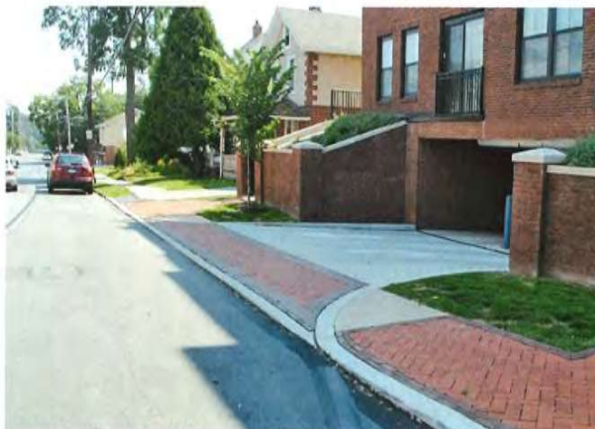
Curb Cut located along the rear of the lot/building
