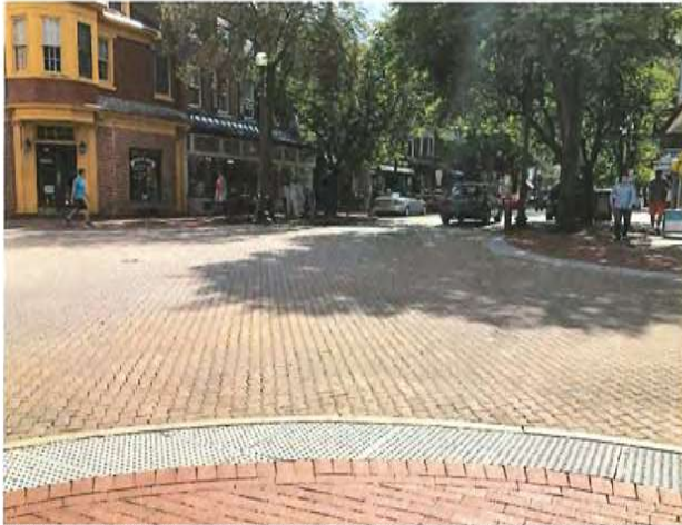
ADA Accessible ramps provided at all street intersections
