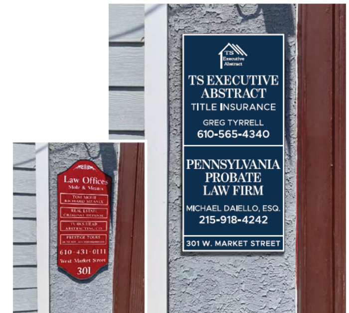
The existing building sign will be removed, and the new sign will be installed in its place with VHB tape and silicone.
