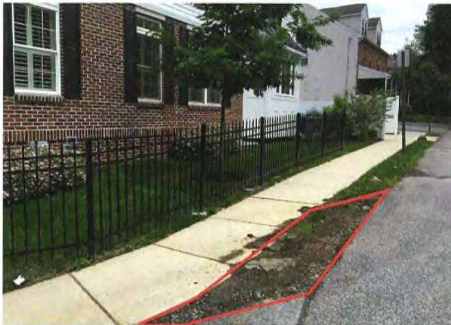
Alley with Grass Edge Problem that could be converted to River-Jack Stone
