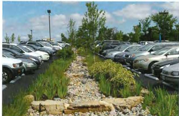
Off-Street Parking landscaped with the incorporation of LID practices
