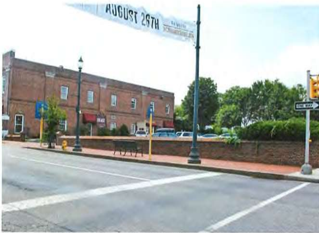
Street Wall utilized to screen Off-Street Parking located at a corner location
