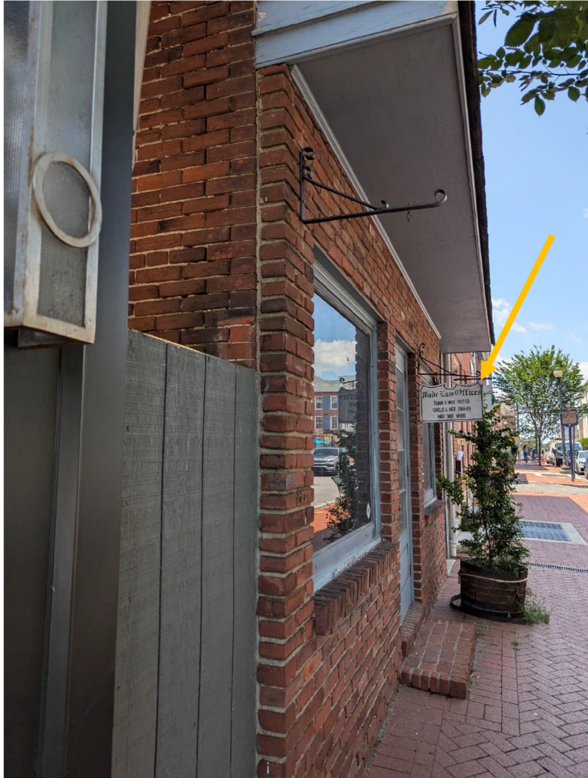
Current view from sidewalk- brick step 24 inches (pic. 1)
