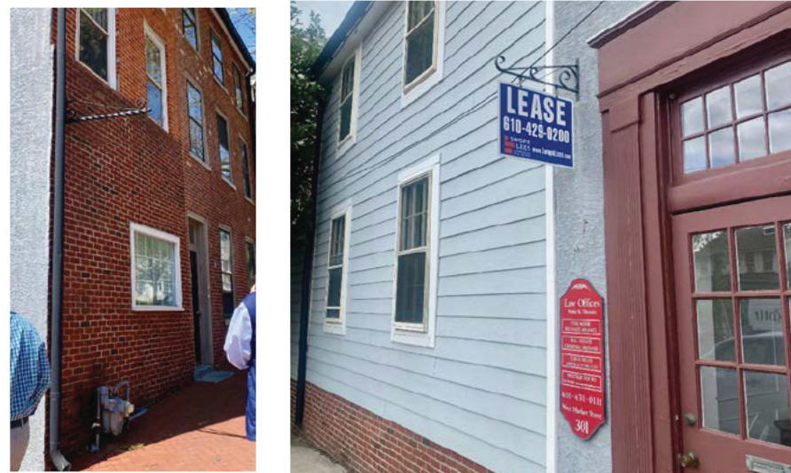
The new signs will be mounted to existing scroll brackets with new stainless steel hanging hardware. The larger hanging sign will be secured with an additional new scroll bracket at the bottom to prevent swinging.
