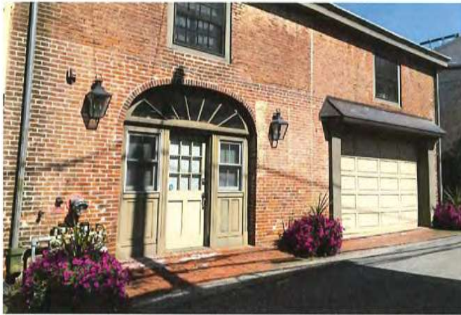
Well Designed Facade with Side Lights to Front Door, Fan Light above Front Door, and Pent Eave Roof above Garage Door
