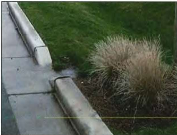
Curb Openings allow rain water to enter bioswale for infiltration
