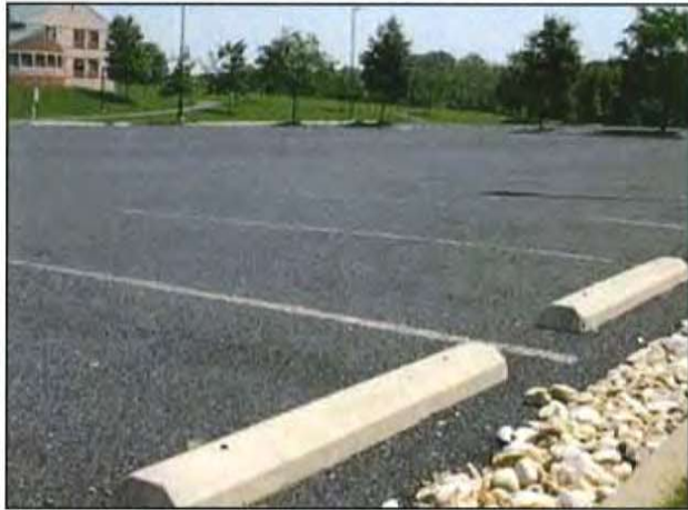
Parking Lot Stone Edge to slow down runoff and allow infiltration
