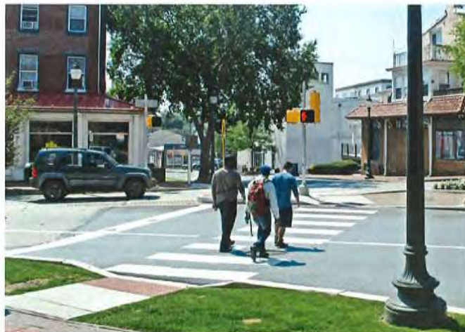
Crosswalk Striping connecting opposing accessible sidewalk ramps
