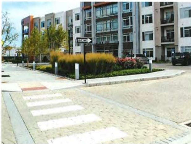
Concrete pavers and Belgian Block curbing used to enhance parking court
