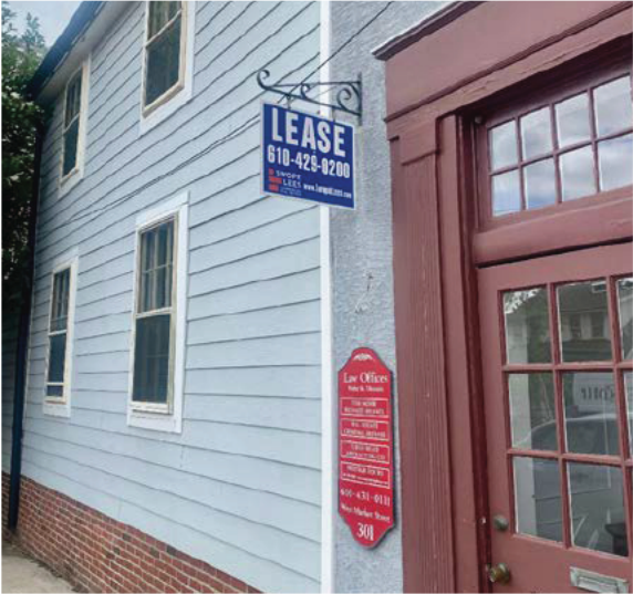
The new signs will be mounted to existing scroll brackets with new stainless steel hanging hardware. The larger hanging sign will be secured with an additional new scroll bracket at the bottom to prevent swinging.
