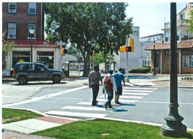
Crosswalk Striping connecting opposing accessible sidewalk ramps
