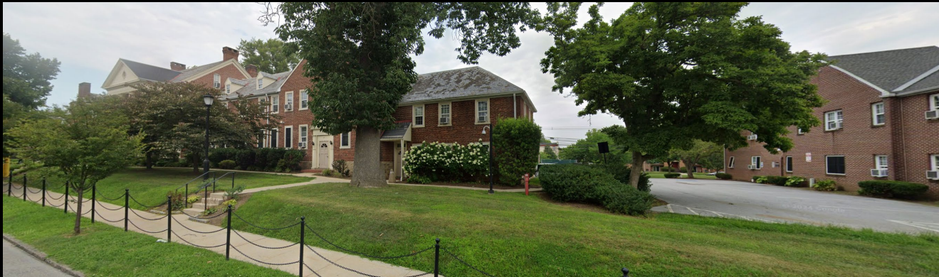
S. High St (East and North Buildings)
