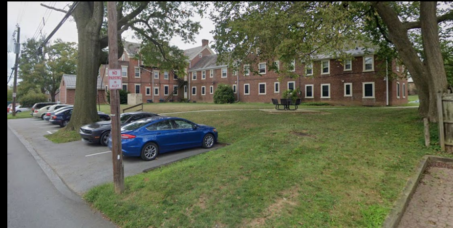
Sharon Alley – Rear view (North Building)
