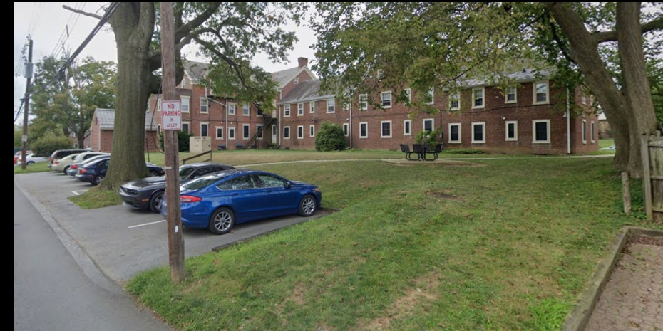
Sharon Alley – Rear view (North Building)
