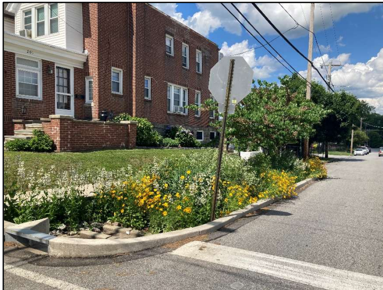
Figure 2 – Sample Rain Garden Curb Bump-out at Chestnut Intersection
