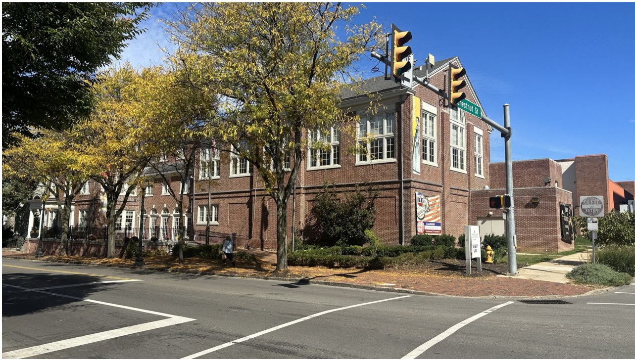
01 CCHC - LOOKING NORTHEAST S1
